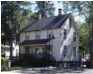
Cottage at 171 Henry St
