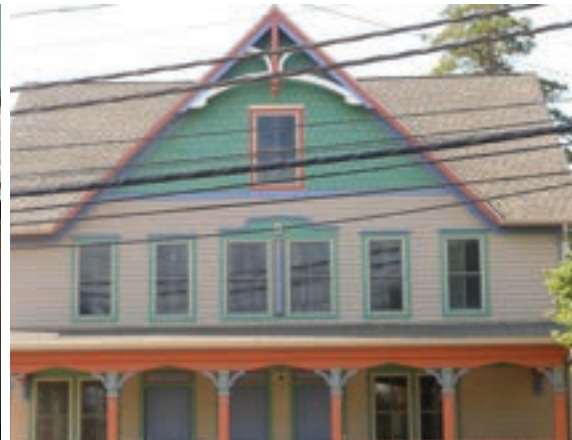
LIGHTHOUSE I STAMFORD OPENED: 2018 INDIVIDUAL UNITS: 9
