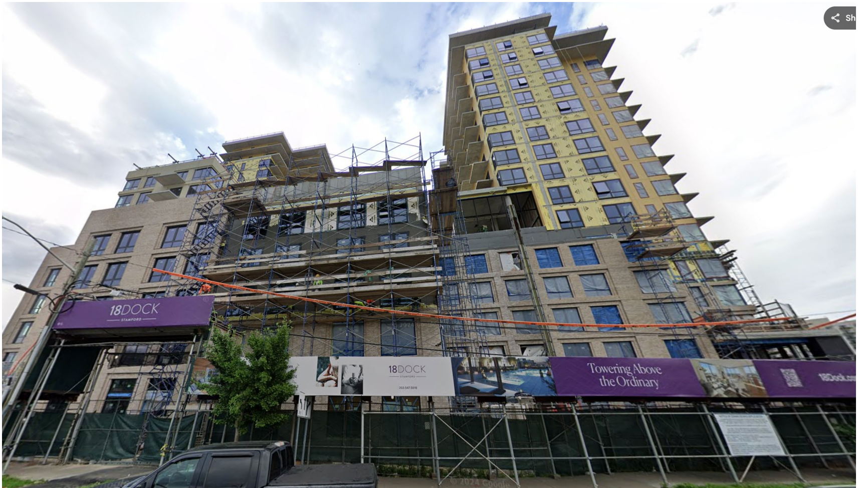
18 Dock St. shown above had 395 units
