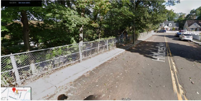
Looking east to intersection of Hillcrest Avenue and Lindale Street
