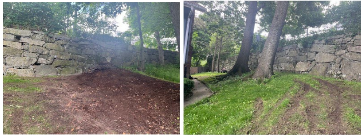
Retaining Wall along Hillcrest Avenue (view from 54 Underhill Street)
