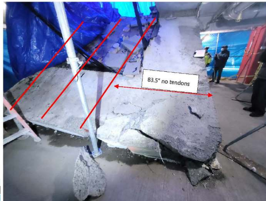
Figure 10- PT Layout at Slab Looking East to West
