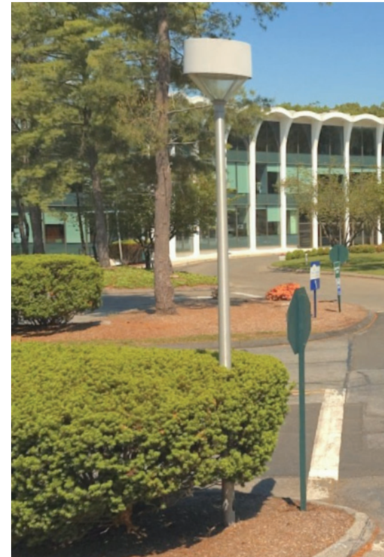
POLE TOP LUMINAIRE WITH INDUCTION LAMP
