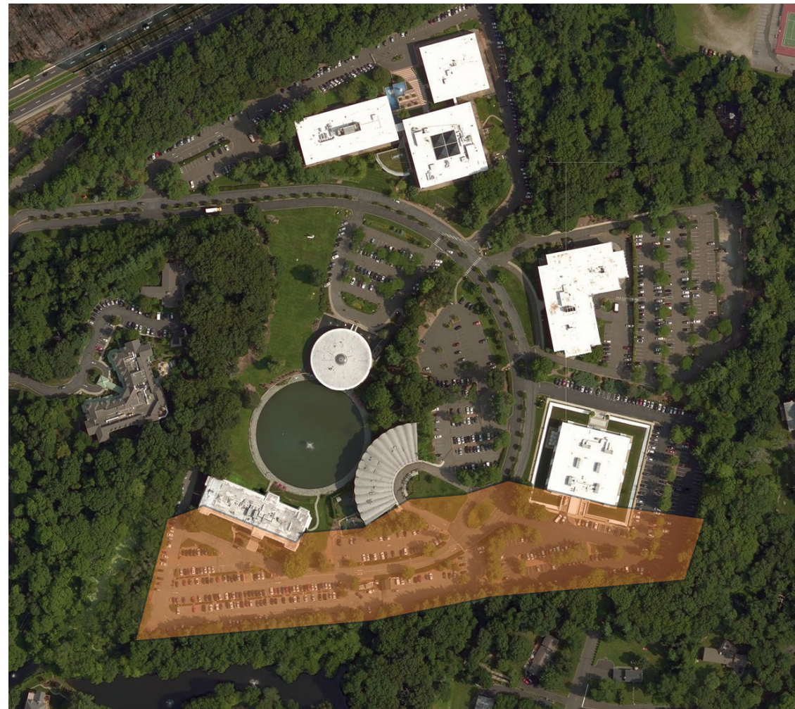
SITE PHOTOGRAPH OF HIGH RIDGE PARK SHOWING SURVEYED AREA
