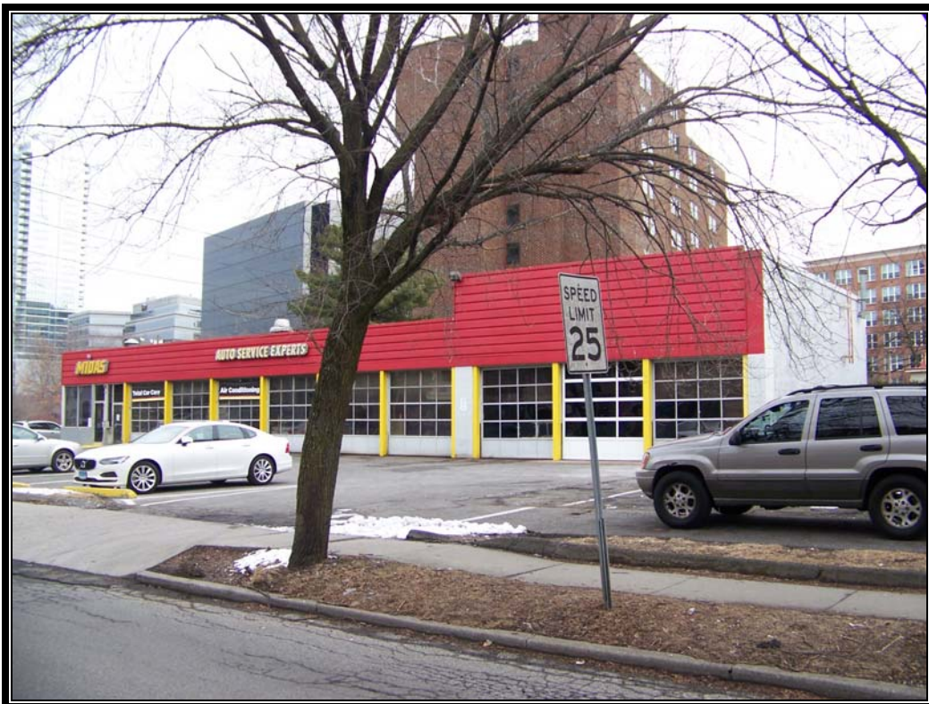
Front and side view of improvement
