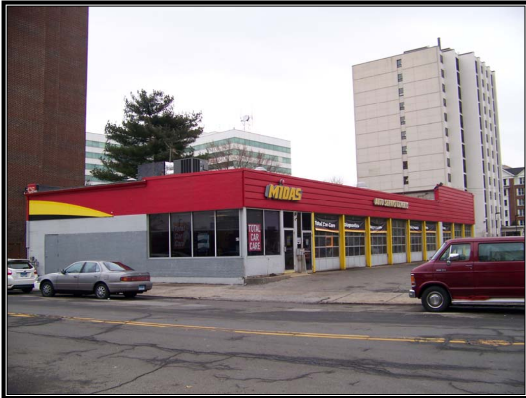
Front and side view of improvement
