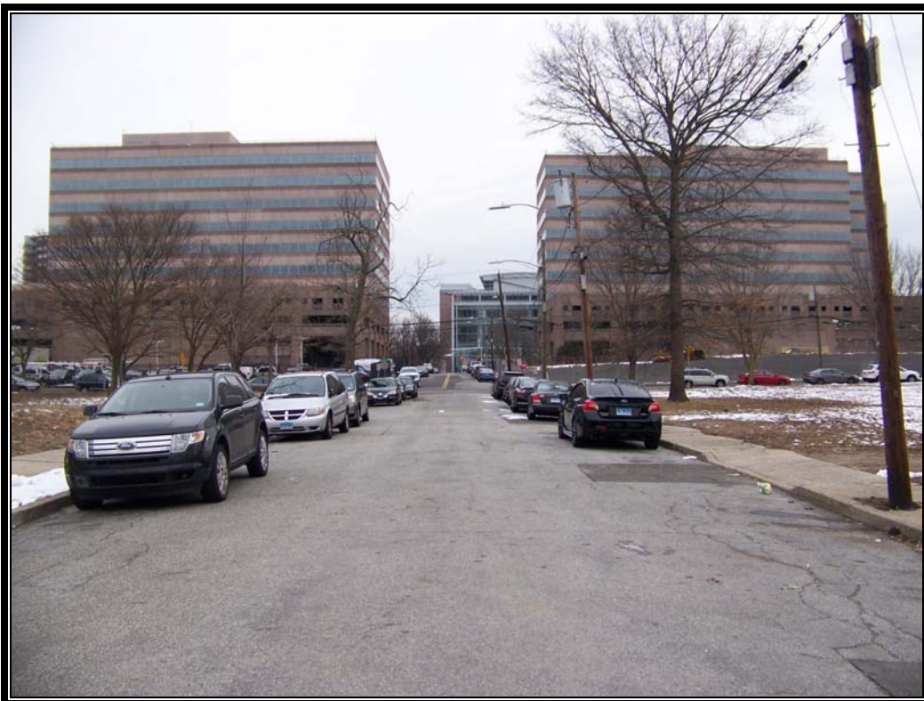
Easterly view of roadbed of Division Street (west of Clinton Avenue)
