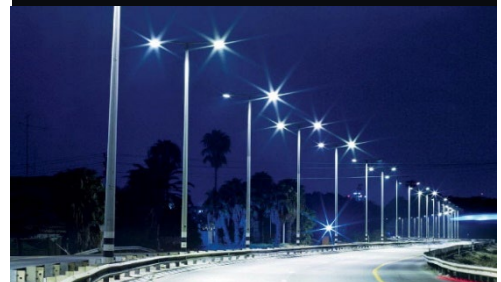
LED Street Lights
