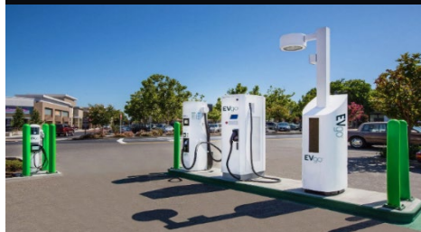
Electric Vehicle Charging Stations
