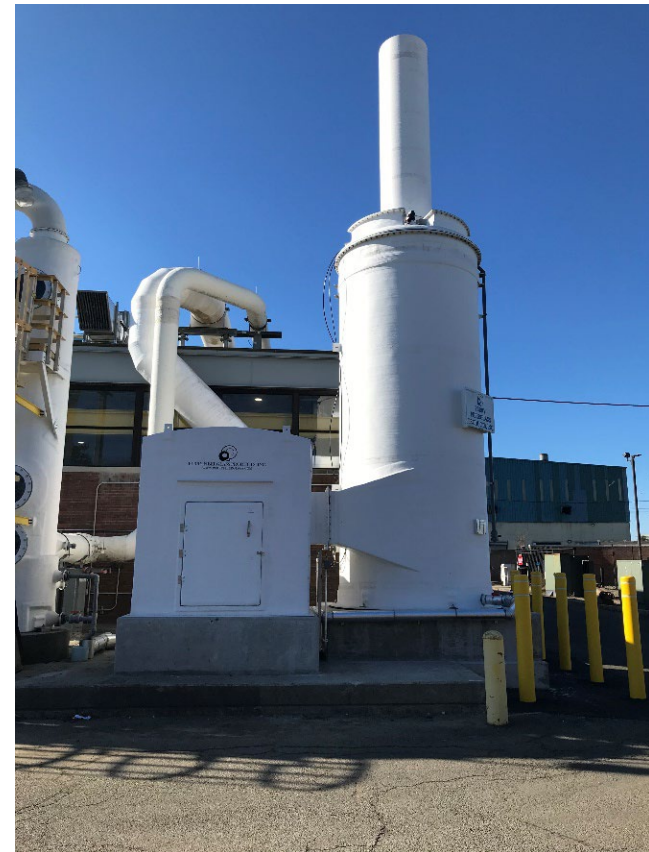
New Odor Control
