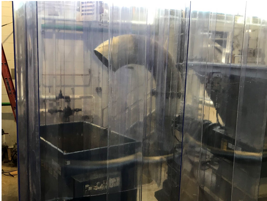
New Screenings Grinder, Washer, Compactor
