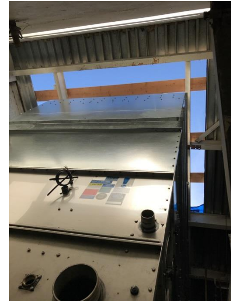
1 of 3 Cooling Sections being installed
