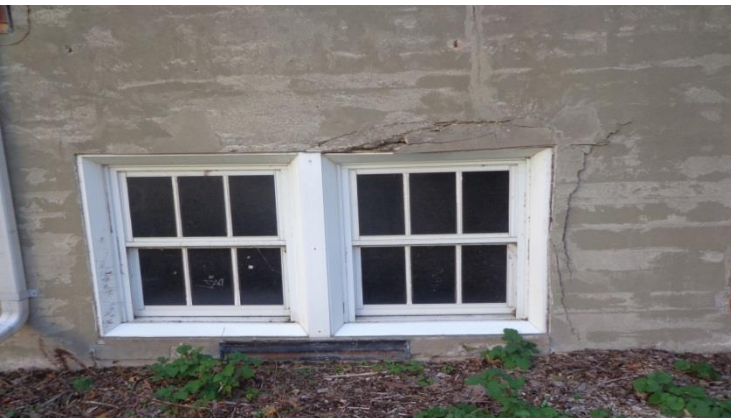
Failing Foundation Wall in the North Interior Courtyard
