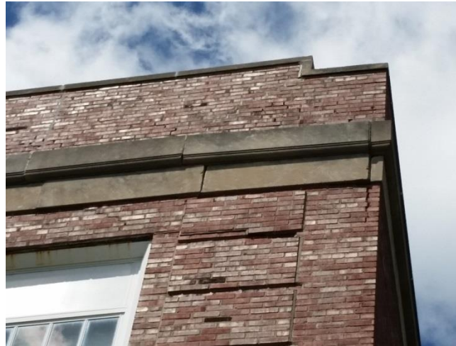
Structurally Unstable Parapet Wall at Northeast Corner of the 1927 Building
