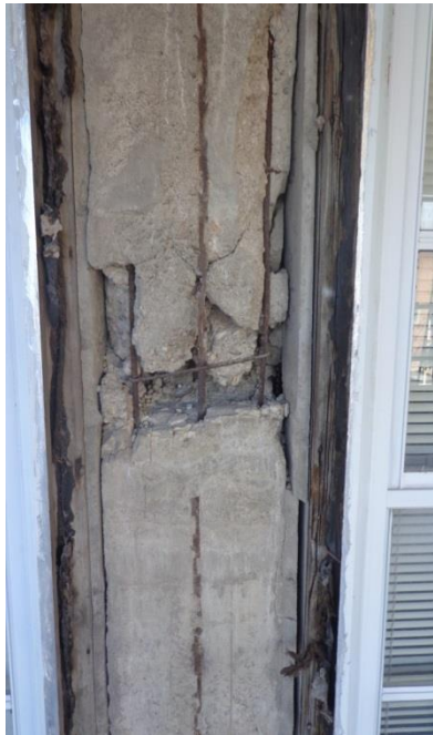
Structurally Unstable Column. Exposed & repaired once brick façade was removed.
