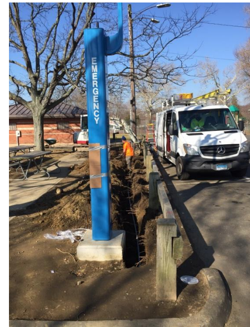
Present Condition at Lione Park (March, 2016)
