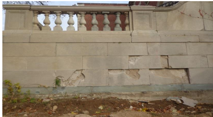
Crumbling Limestone Façade, Auditorium Main Entrance
