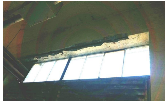
Interior Concrete Head of Masonry Opening Above (with structural cracking)
