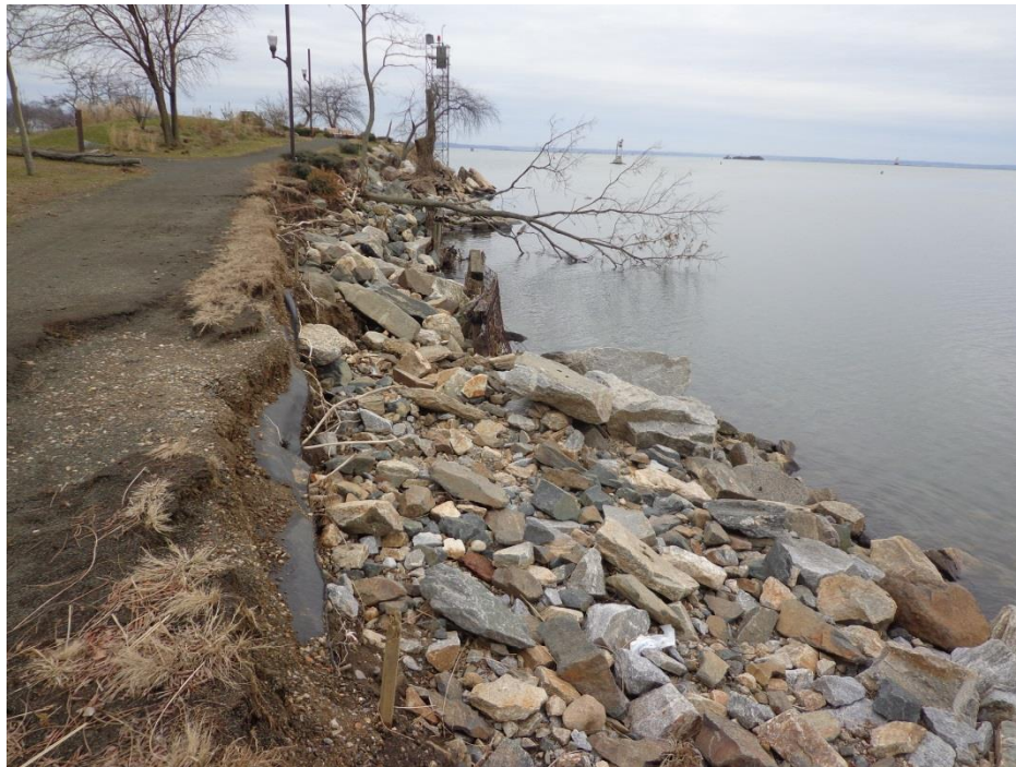
Condition After Sandy Storm
