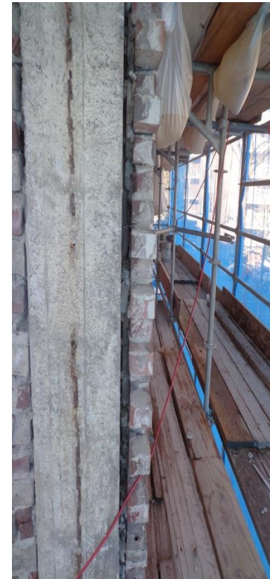
Existing Brick Façade Pulling Away From Back-up Structure
