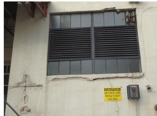
Failing Foundation Wall at Loading Dock
