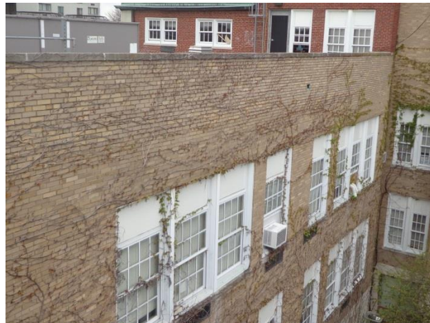
Structurally Unstable Parapet Wall at Northeast Corner of the 1927 Building
